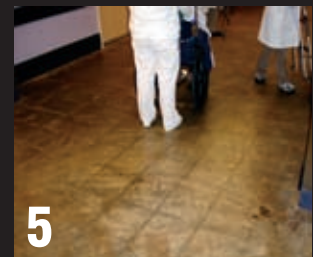
4. Crewman install a concrete moisture sealer on a new slab at a Southern Californian high rise hospital building. 5. A floor failure with missing tiles in a Northern California hospital caused by concrete slab moisture.
